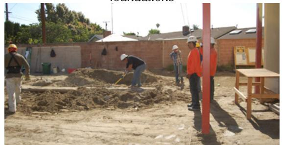
*Using sledgehammers to break concrete footing*
